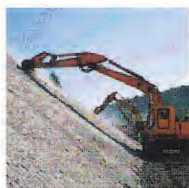
Cutting face of slope
