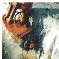
Chipping the concrete surface
