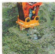
Digging the foundation for electric power pylon
