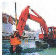
Cutting the bottom of dam
